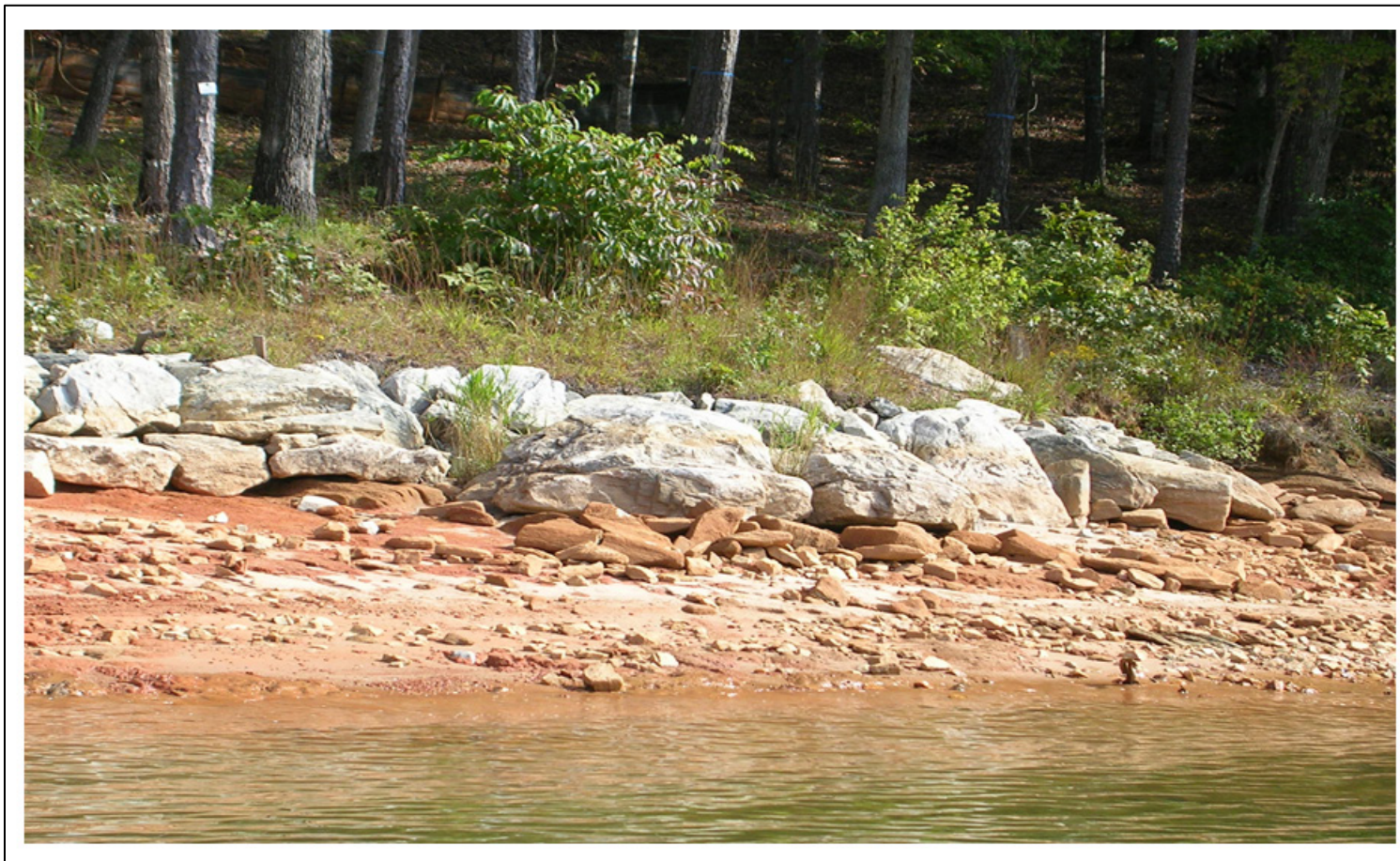
Figure 23. Enhanced Riprap (with Boulders and Plantings)
